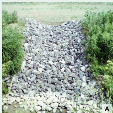
Photos 1 A and B : Rock chute spillway Source : Bernard Arpin and Robert Beaulieu (MAPAQ)
