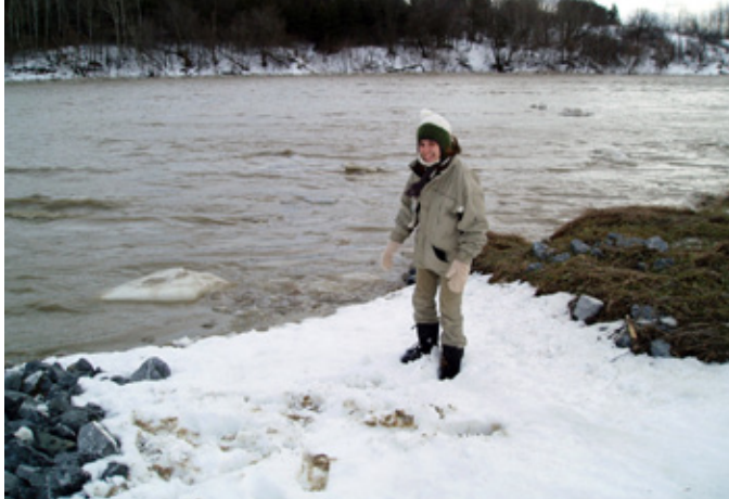
Photo 6 : Rock chute spillway on the bank of the Yamaska River Source : Ghislain Poisson (MAPAQ)
