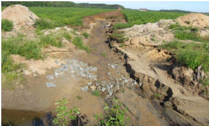
Photo 12 : Downcutting (Inlet apron too short and too low relative to the bottom of the furrow) Source : Victor Savoie (MAPAQ)
