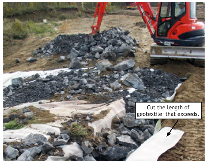
Photo 8 : Anchor trench of inlet apron Source : Mikael Guillou (MAPAQ)
