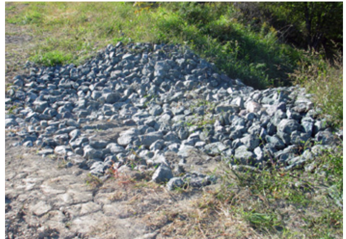
Photo 10 : Placing riprap Source : Victor Savoie (MAPAQ)
