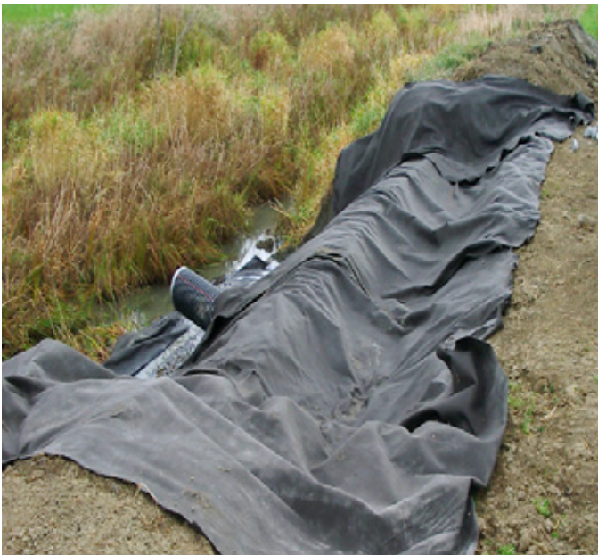
Photo 9 : Installing geotextile Source : Georges Lamarre (MAPAQ)
